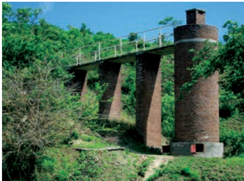
Figure 10. An Example of a Vertical Kiln for Limestone Burning
