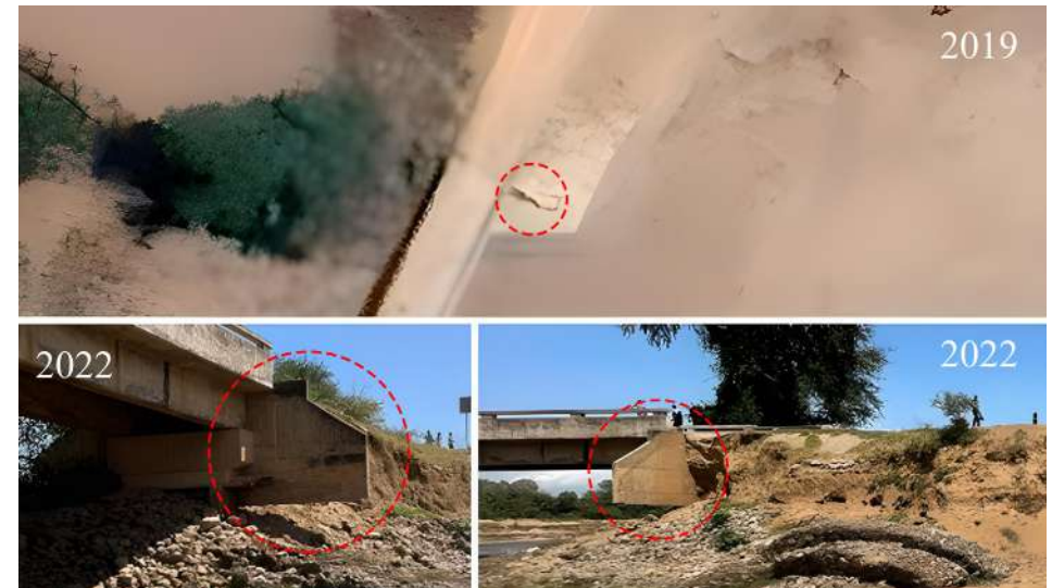
Figure 10- River erosion at the Mwamphazi bridge
