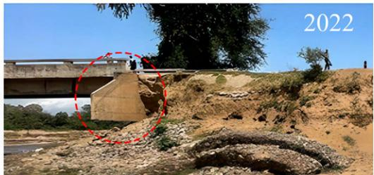
Figure 10- River erosion at the Mwamphazi bridge
